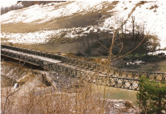
Army bridge replacing one destroyed in the Bosnian war
