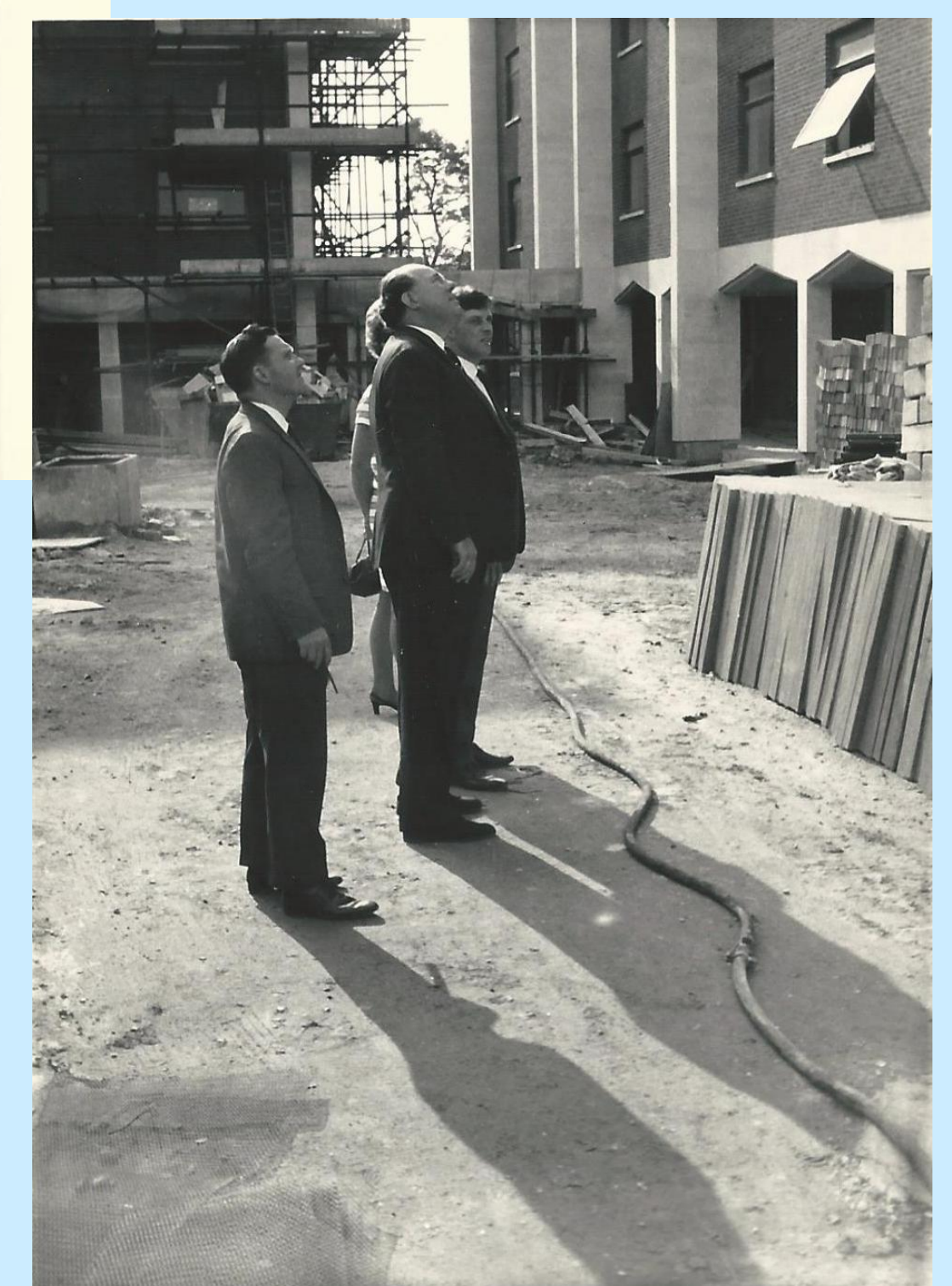
Photographs of Cripps under construction and site visits by Gordon Woollatt, the Architect
