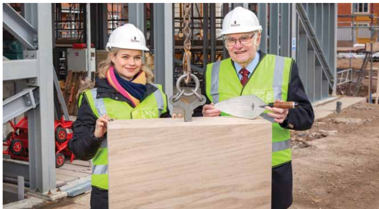
Principal donor, Chris Dobson (SE 1957) and his daughter, Abigail Bennington, lay the foundation stone for the new library and auditorium, 3 rd February 2020.
