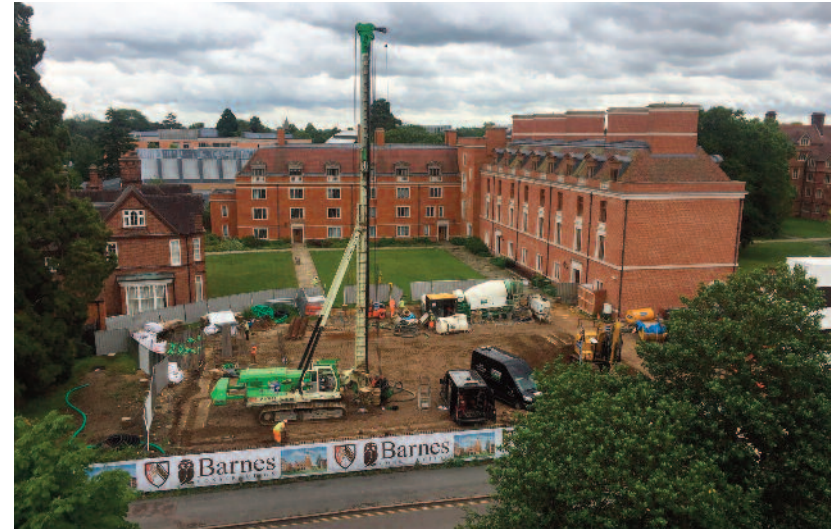
Construction work on the new library and auditorium in June 2019
